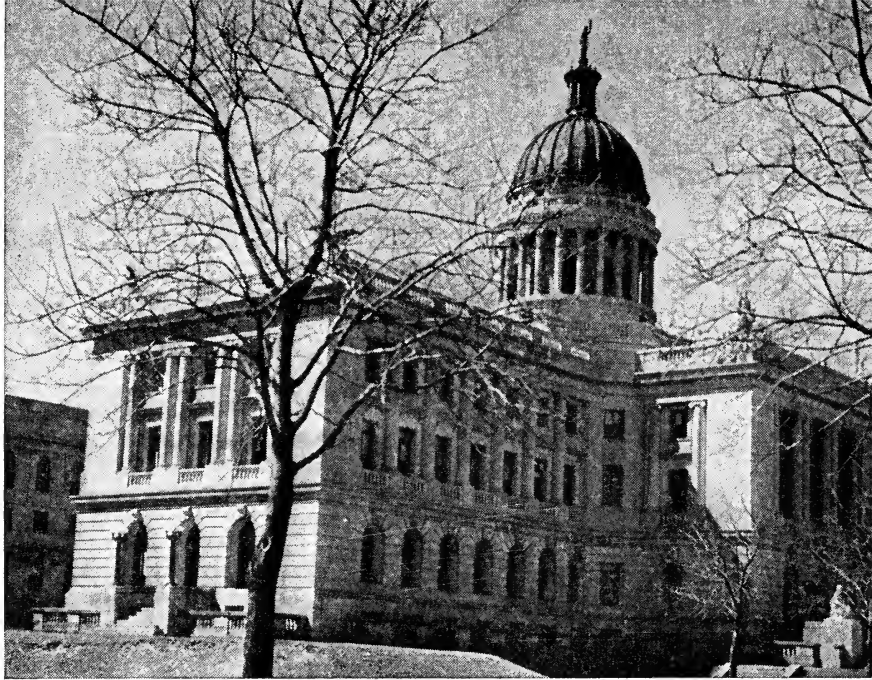
BERGEN COUNTY COURTHOUSE, HACKENSACK
